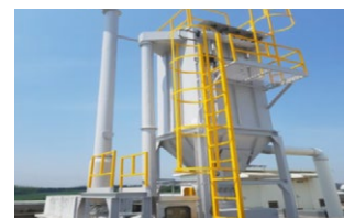
Prevention of fall accidents related to safety scaffolding for dust collection equipment
